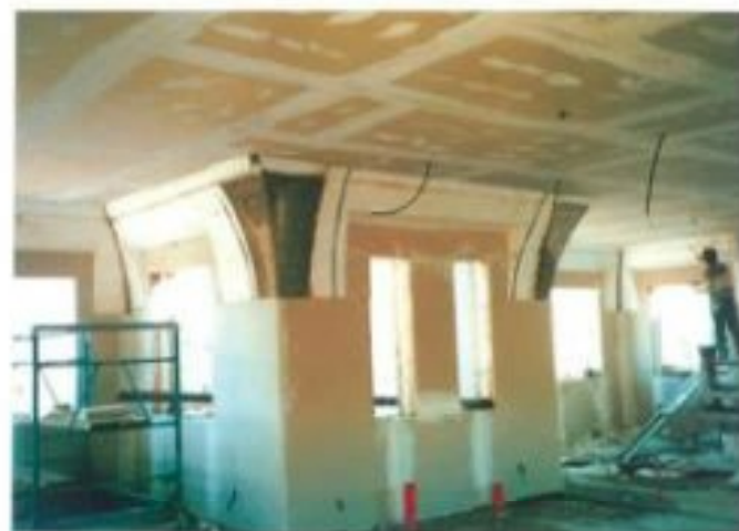
* Realizarea interior cu panouri de carton-gips * Interior furnishing with plasterboard panels
